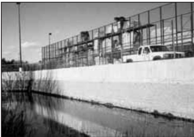
When there is no room to set guide rails behind a wall, traffic barriers can be placed directly on top of a wall.
