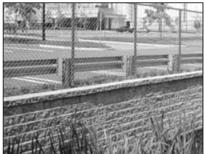
When space allows, fences and railings should be placed several feet behind VERSA-LOK walls.
