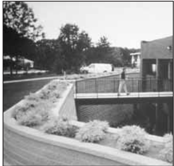
Back-to-back VERSA-LOK walls spaced far enough apart can act as pedestrian barriers while providing room for plantings.
